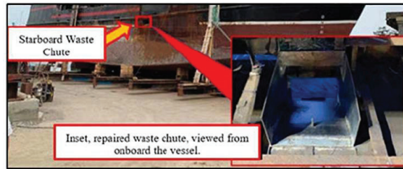
Figure 94 – SCANDIES ROSE on the blocks May 2019 at Lovric's Shipyard, Anacortes, WA. "Starboard waste chute" highlighted, with inset photo showing repaired waste chute as viewed from onboard the vessel, looking outboard. Inset photo, lower right, displays the completely rebuilt starboard waste chute as repaired later in 2019 by High Mark Marine certified welders in Kodiak, AK. (Source [redacted])
